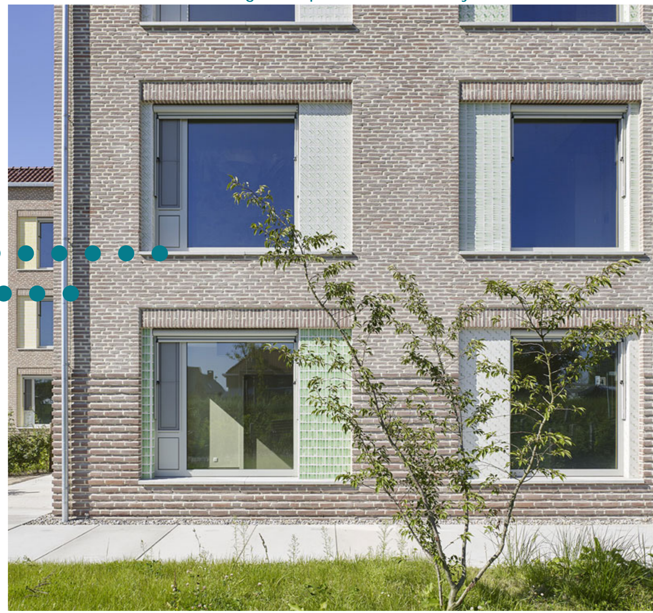
Brick detailing and openable window systems
