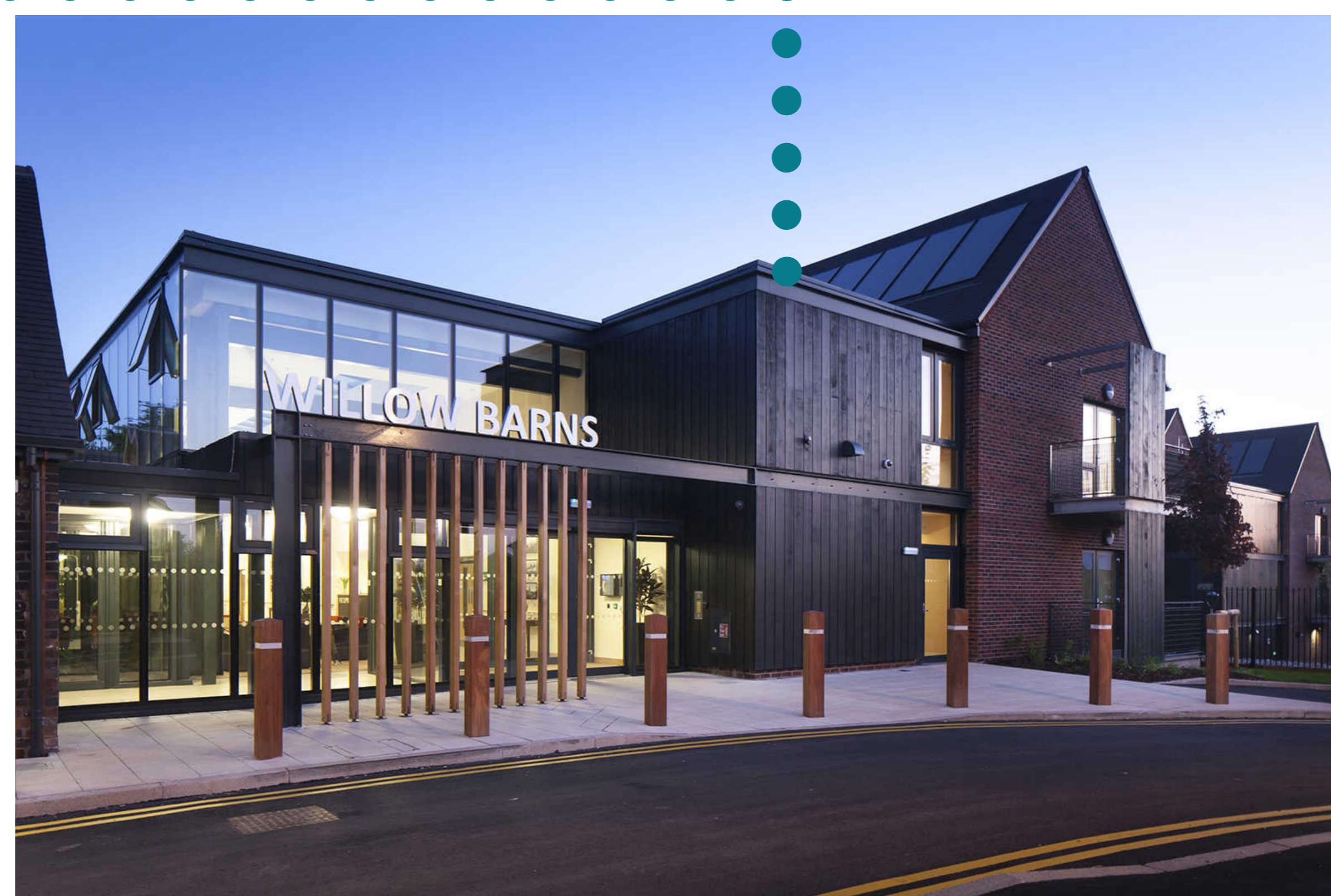
Metal/ darker cladding against lighter materials
