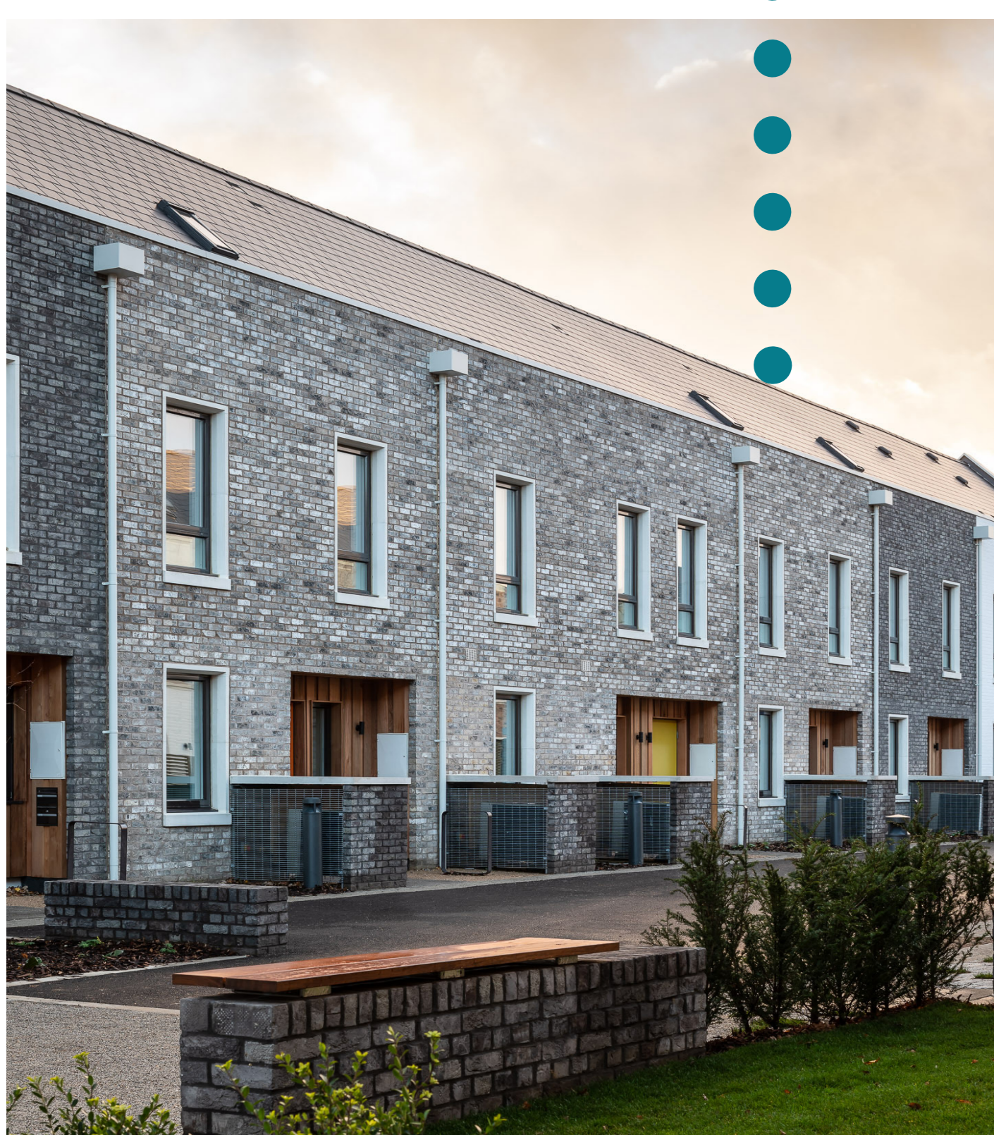
Contemporary slate roof
